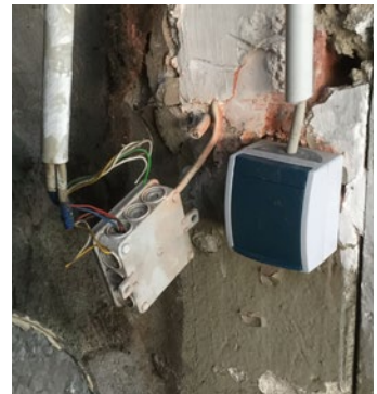
Abb. 6 Defekte Installation
